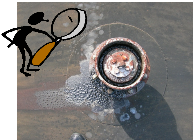
Is a leaking package vent okay? What is protecting the general public from this hazard?
